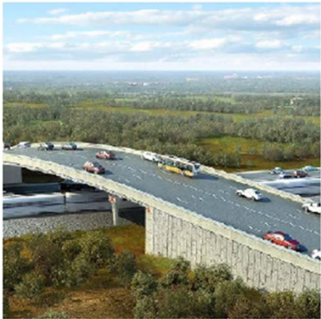
The proposed overpass (above), as part of the Cibolo Parkway Toll portion, would allow drivers and emergency vehicles to drive over FM 78 and the Union Pacific Railroad.
